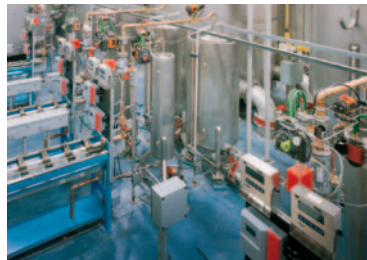
Hydro Lab in Badger Meter's James O. Wright Innovation Center
